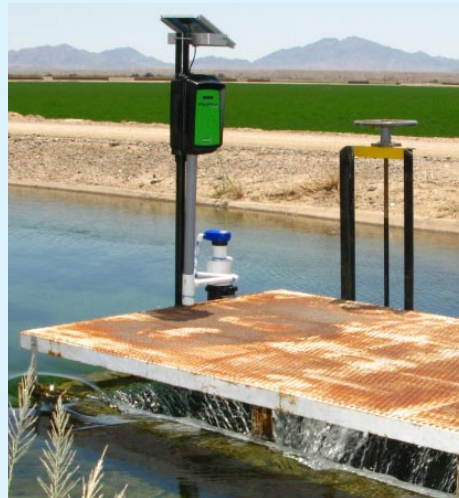
Figure 1: The broad-crested weir structure at Quail Mesa Ranch, AZ.
